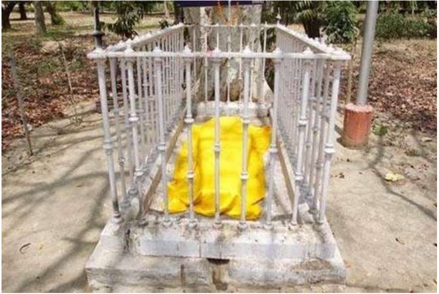
above: Sergeant Watkins' tomb at Allahabad before its recent demolition (see page 49)
