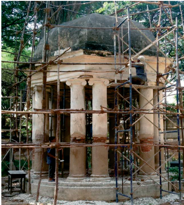
Hyderabad: the Residency Cemetery. Frances Sydenham's tomb. Applying lime mortar to consolidate the columns.
